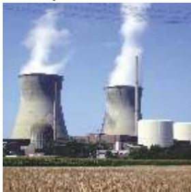
Power & Ash Handling
